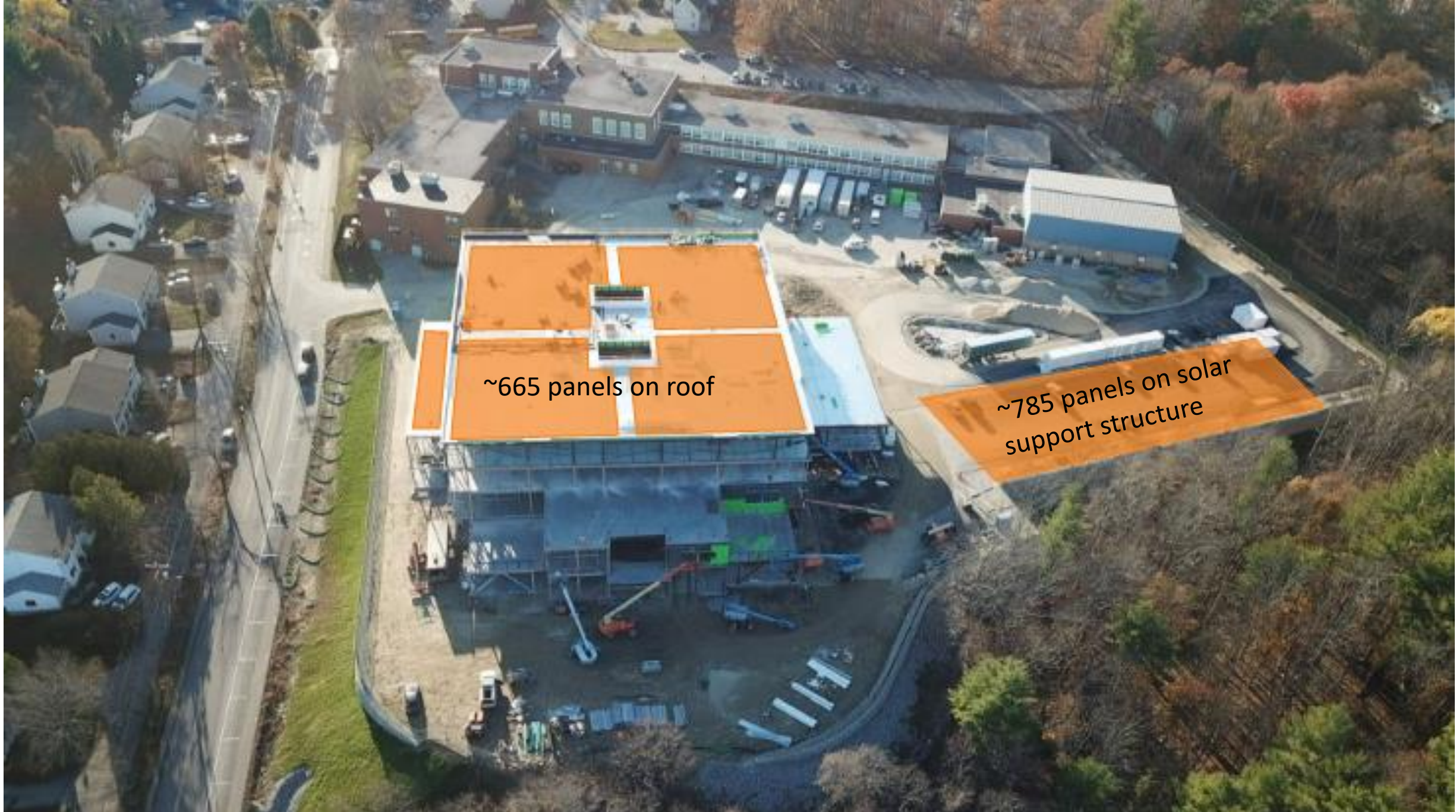
Aerial view of new ORMS construction, early December 2020
